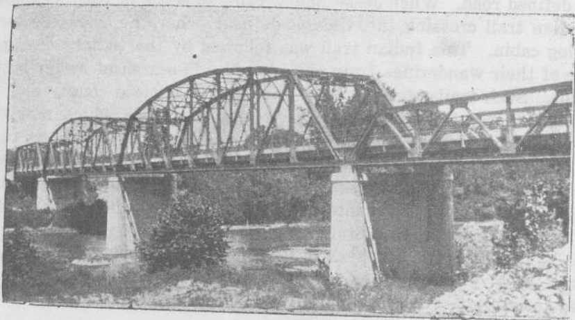
THE BRIDGE ACROSS THE GASCONADE RIVER
