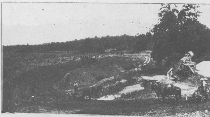
CONSTRUCTION WORK ON A HIGHWAY
