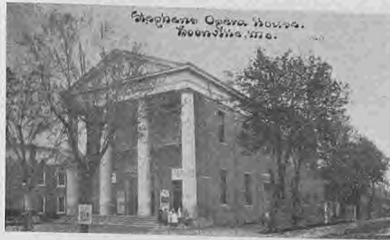
STEPHENS OPERA HOUSE, BOONVILLE, MO.
