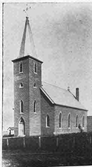
EXTERIOR VIEW OF MARTINS- VILLE CATHOLIC CHURCH, R. F. D. No. 3, BOONVILLE, MO.
