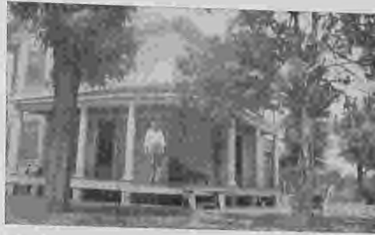
RESIDENCE OF L. V. WENDLETON, This Residence is shown partially completed. It is being built at a cost of $7,000 00. It is constructed with native hard lumber grown, sawed and milled on Mr Wendleton's own farm. SPEED, MO.
