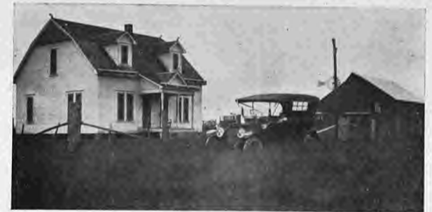
RESIDENCE OF EDGAR A. CARPENTER, BUNCETON, MO.
