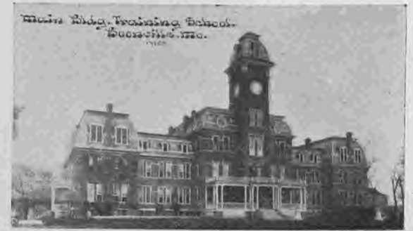
MAIN BUILDING OF TRAINING SCHOOL, BOONVILLE, MO.
