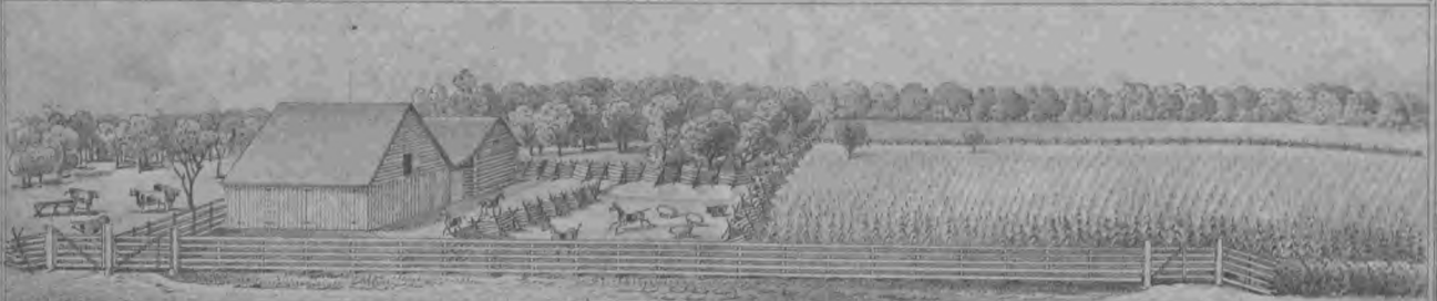
LOOKING NORTH FROM THE HOUSE
